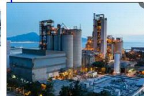
Nitrogen Fertilizer Plant: 450 tonne/day
