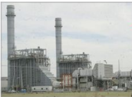
Gas Turbine, powered by Hydrogen
