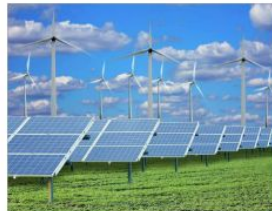
Purpose-built Solar & Wind 200 MW PV on 1200 acres
